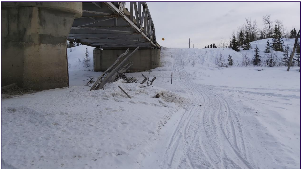
Figure 3. Wood accumulation on the upstream side of the pier under the Alaska Highway bridge on the Takhini River. The photo is looking towards the right bank where the station is located.
