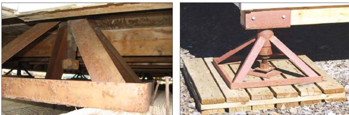
**Figure F11.** Examples of adjustable-jack foundations from Gravel (2012) and CSA (2010).
