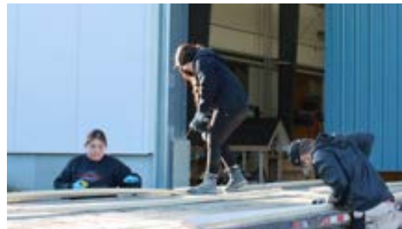
Students assisting to crib house onto trailer.
